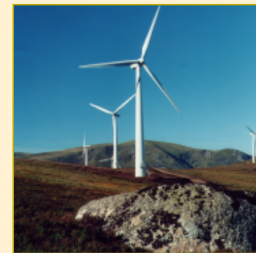
Novar Wind Farm, Ross-shire, Scotland Photo © npower renewables 2005
